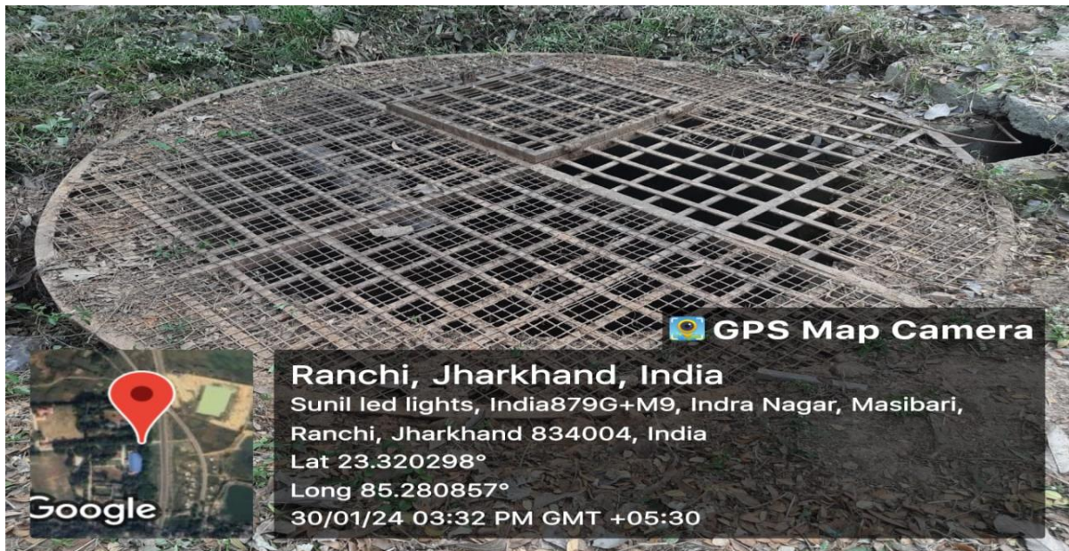
Rain Water Harvesting
